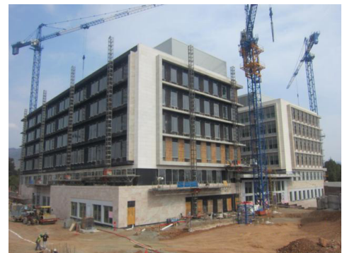
Construction Photos - U.S. Department of State
