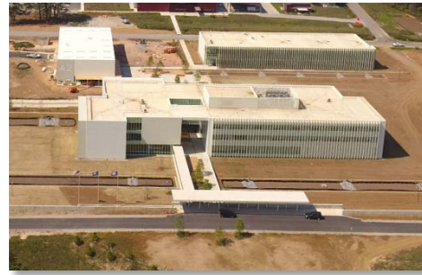
Photo Left: Completed Administrative and Classroom Building in the foreground and the Tactical Training Building venue behind it on the right side.
