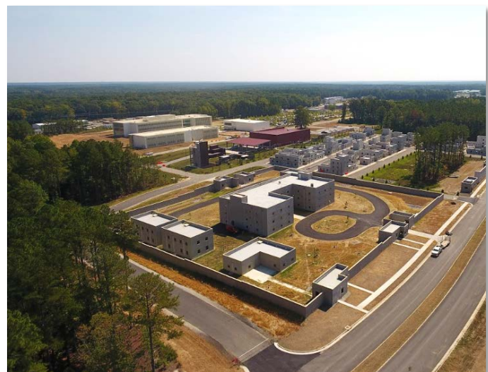
Photo Above: Located at the forefront and center is the completed Mock Embassy training venue from Contract 02.
