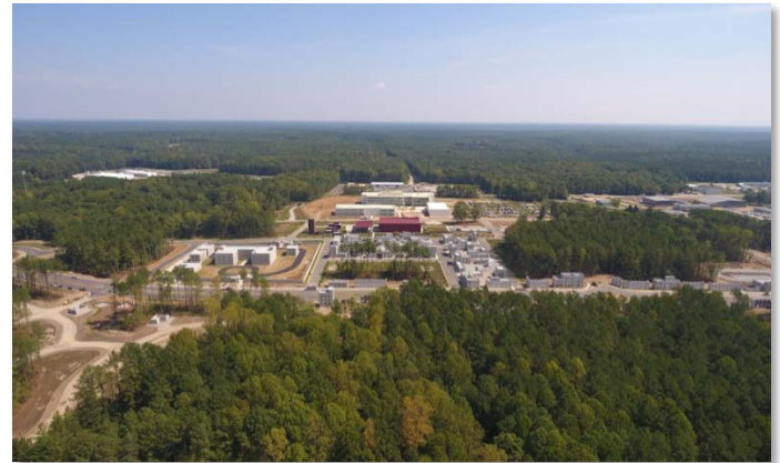
Photo Above: Numerous FASTC training venues from all three construction contracts.
